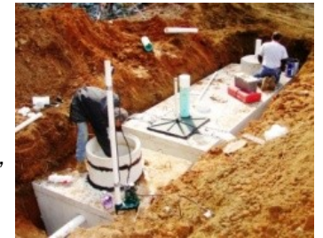
A FAST (Fixed Activated Sludge Treatment) septic system to reduce nitrogen through multiple biological, bio-chemical, and physical processes
