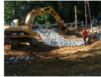
Construction of septic system piping drilled under county road to pump wastewater to upper lot for protecting waterfront groundwater from contamination
